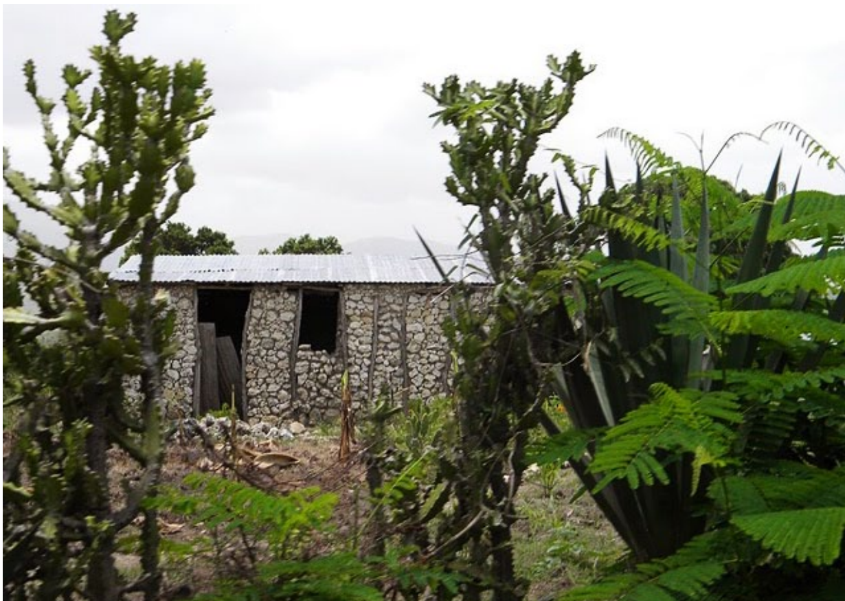
Rural Housing - this dwelling is en-route to the Bois L'Etat site, up in the mountains. Constructed using local rocks found nearby, wood framework, and an aluminum roof.
