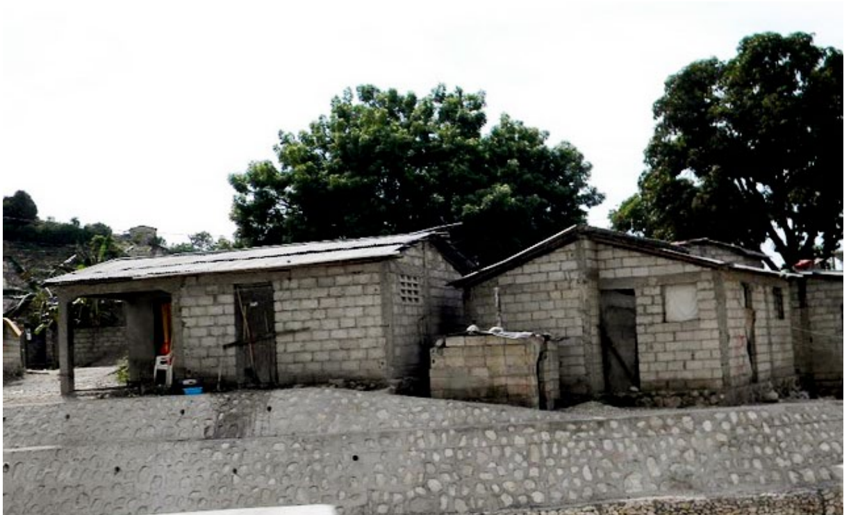
Typical CMU construction with aluminum roofing - however, most houses are finished with some sort of plaster or stucco and painted brightly.
