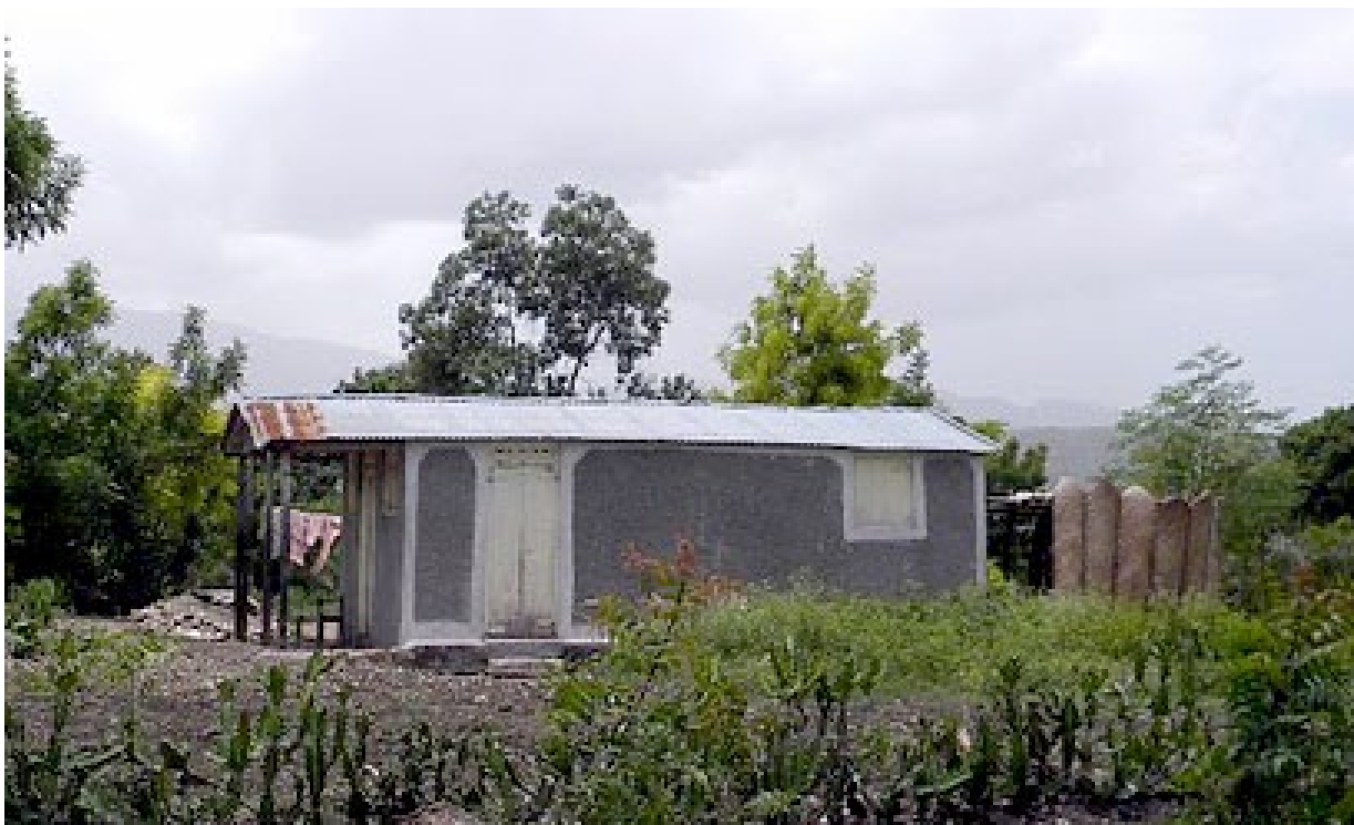
Another rural home en-route to the Bois L'Etat site. Appears to be CMU construction with aluminum roofing.
