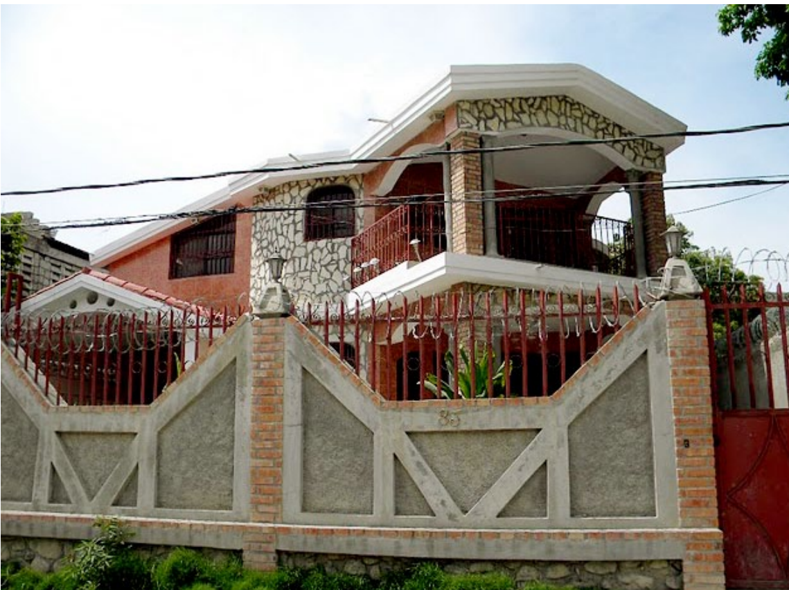
One of the more properly maintained homes in St. Marc - it appears to be of newer construction.
