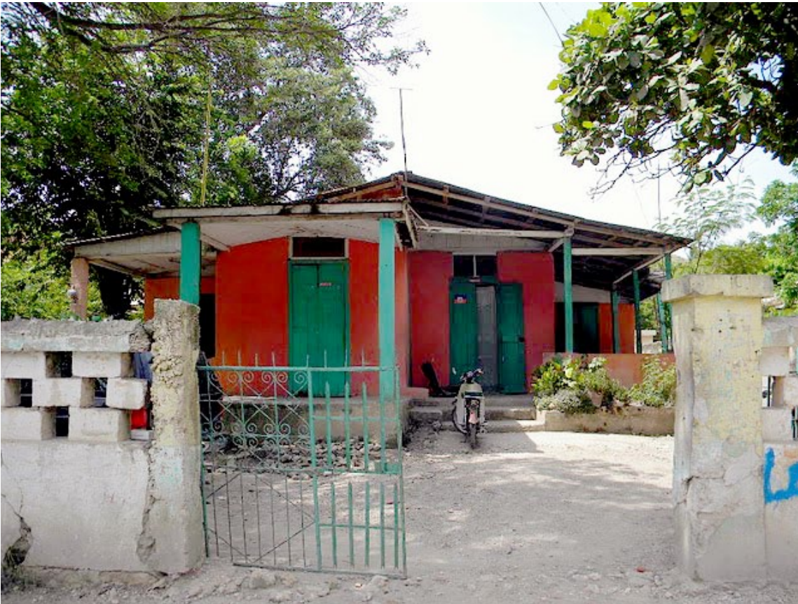
A more “suburban” house (it has a large gated yard and adequate space) in CMU construction with wooden posts and beams and aluminum roof
