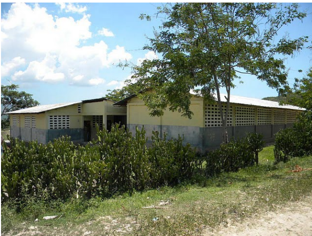
School house .5 km east of Bois L'Etat
