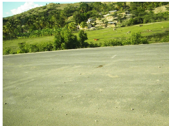
Route 1: after construction
